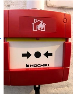
Step 5 Lower section of call point separated with test key still in place.
