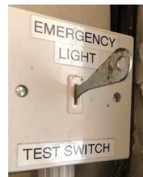
Step 2 Test key angled upwards in “active” position
