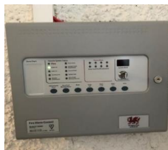
Step 1 Fire Alarm Control Panel - Normal Status
