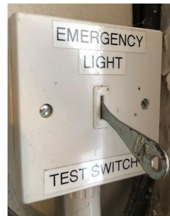
Step 1 Starting position, test key inserted into test switch
