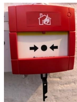
Step 4 Test key inserted into call point
